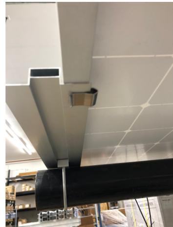
c. Finish the installation with the four (4) clips per module.
