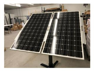
b. Install the second Panel with two (2) clips per side 1.0-3.0" from either end of the purlin as shown.
